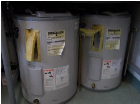
There are two under-counter electric water heaters, but one doesn't work, and there is never enough hot water.
